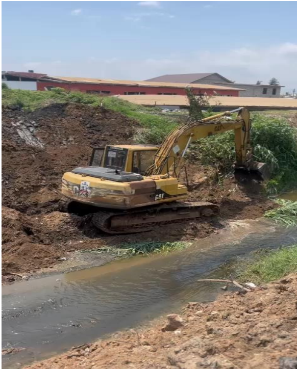
Dredging work on the sections of the Blekese stream
