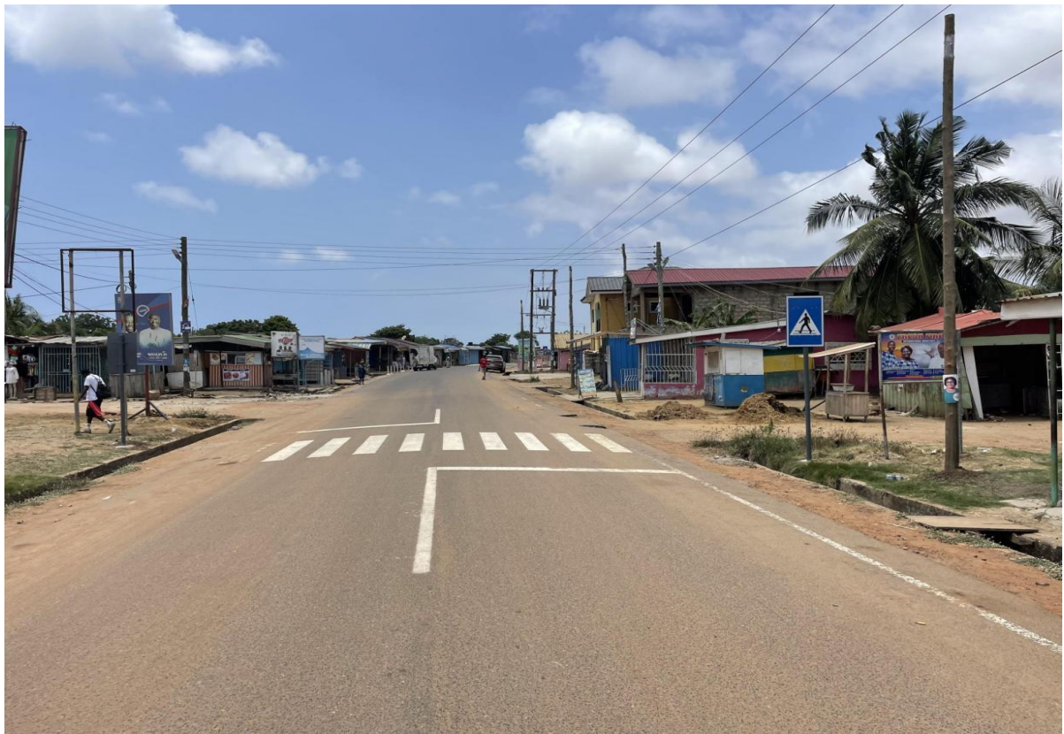
Road safety sign posts, before and after
