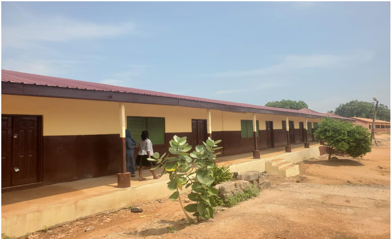
Rehabilitated and renovated of Nungua Methodist '2' Primary School
