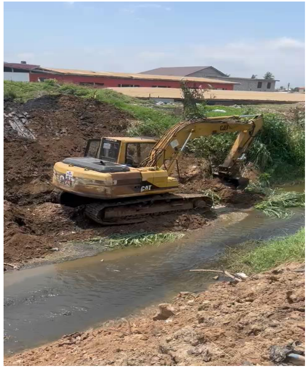
Dredging work on the sections of the Blekese stream
